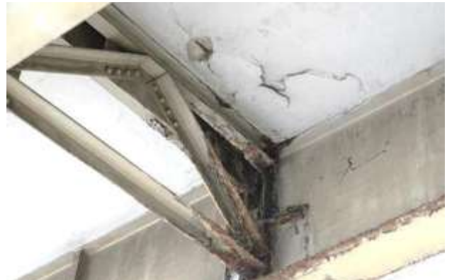
Fig 3.6.3 Warren truss, Rigid joint connection.
