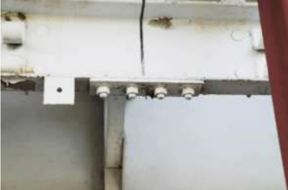
Fig 3.5.4 Rigid joint close up view.
