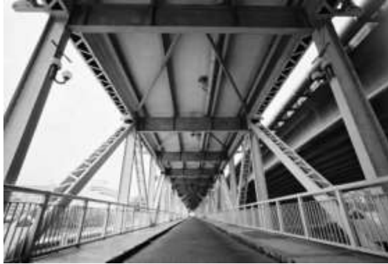
Fig 3.4.1 Interior view of the bridge.
