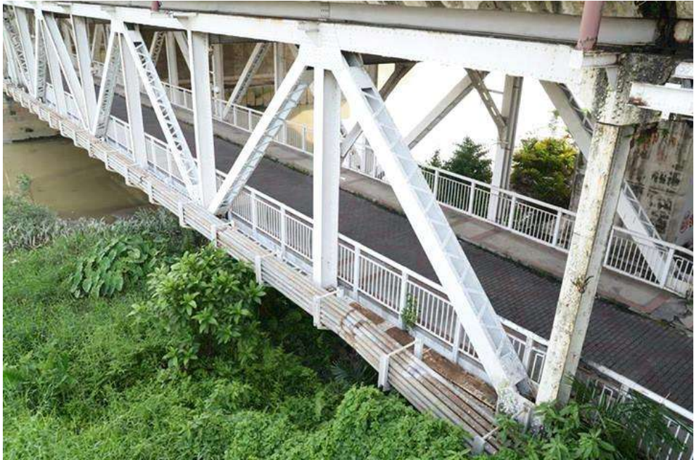
Fig 3.5.1 Overall view of truss connection and members from exterior of bridge.
