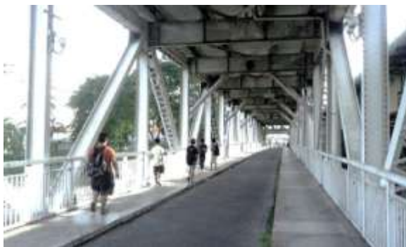
Fig 3.4.3 Interior view of the bridge.
