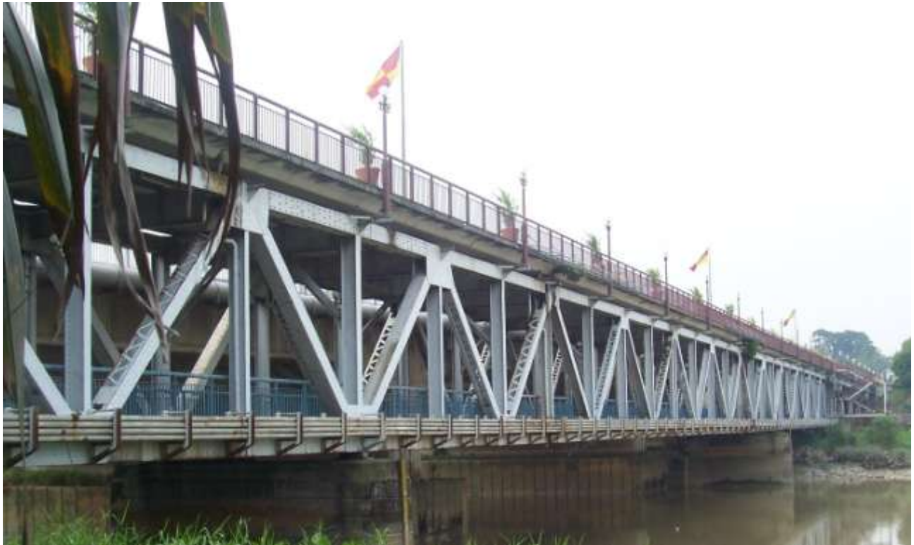
Fig3.1 Exterior view of the bridge
