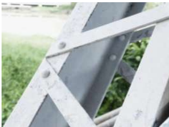
Fig 3.6.4 Pin joint connection, Warren truss arrangement.
