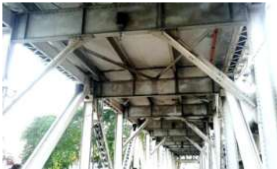
Fig 3.4.2 Interior view of the bridge.
