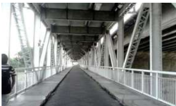
Fig 3.4.4 Interior view of bridge
