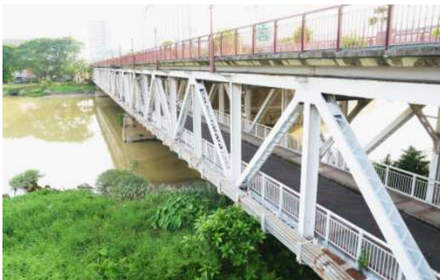
Fig 3.3 View from one side of Kota Bridge
