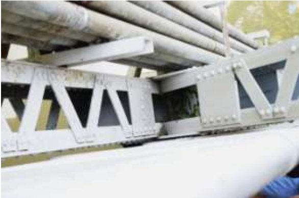
Fig 3.5.2 Rigid joint connections, Warren arrangement
