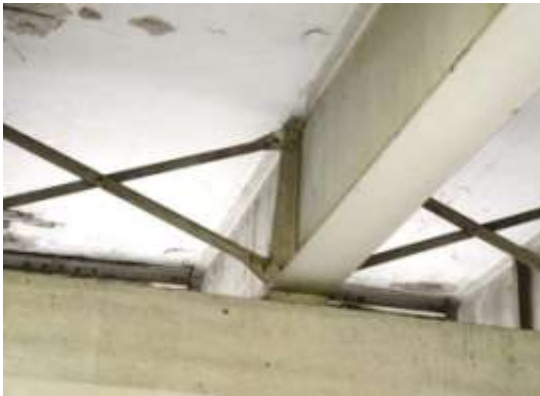
Fig 3.6.2 Double intersection of Warren truss.
