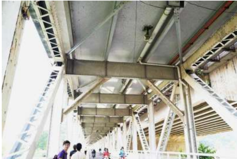
Fig 3.6.1 Overall view of truss arrangement from interior view of the bridge.
